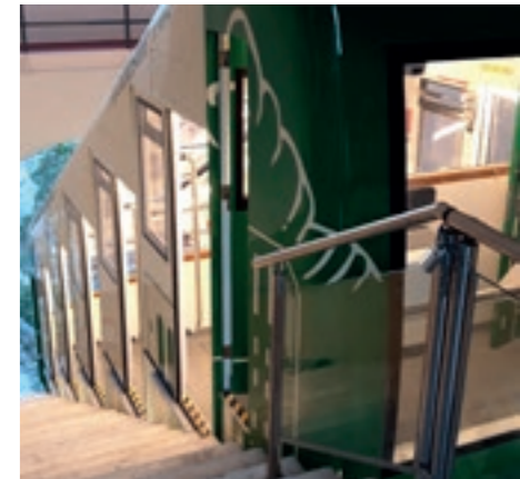
LEITNER SpA – Telefericos Y Nieve - Compoceal AL Cable car -work in progress
