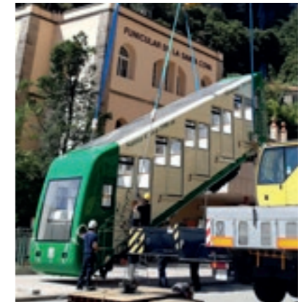
LEITNER SpA – Telefericos Y Nieve - Compoceal AL Wagon at cable car lift departure
