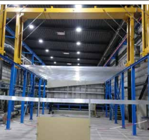
COIL GmbH Bernburg, Germany
